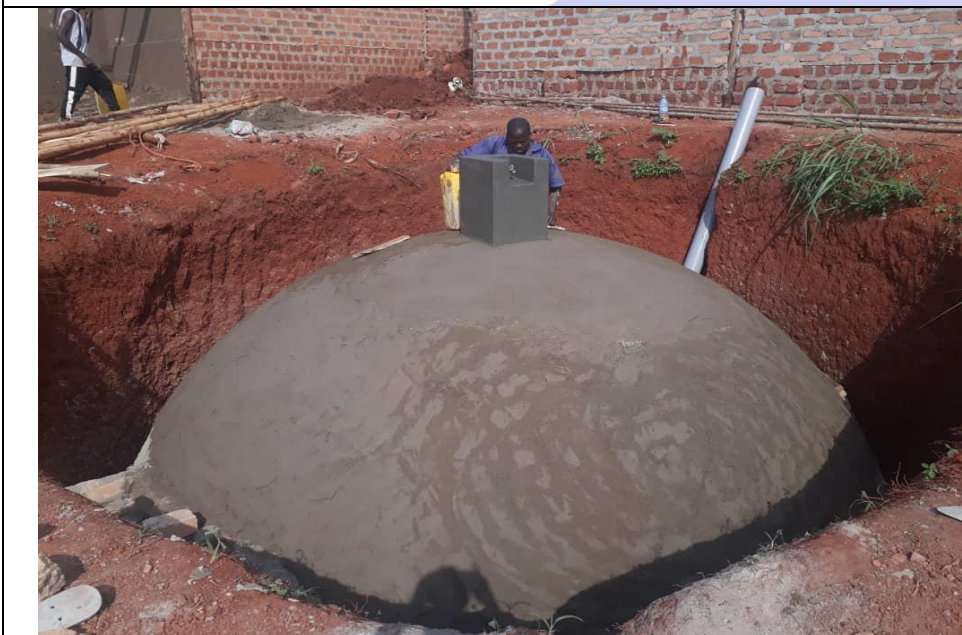
Installed biogas units ready for use
