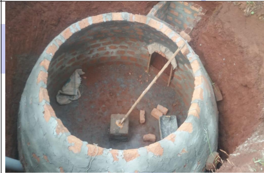
Top view of biodigester under construction
