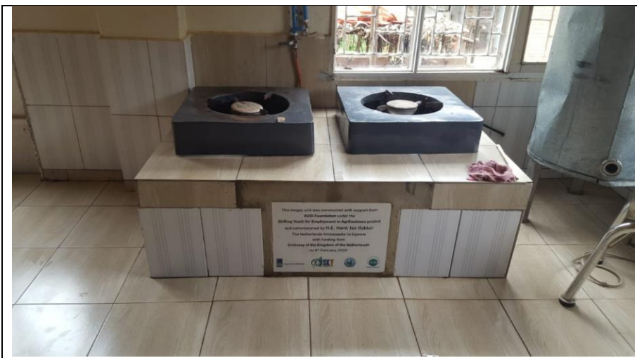
Installed biogas units ready for use
