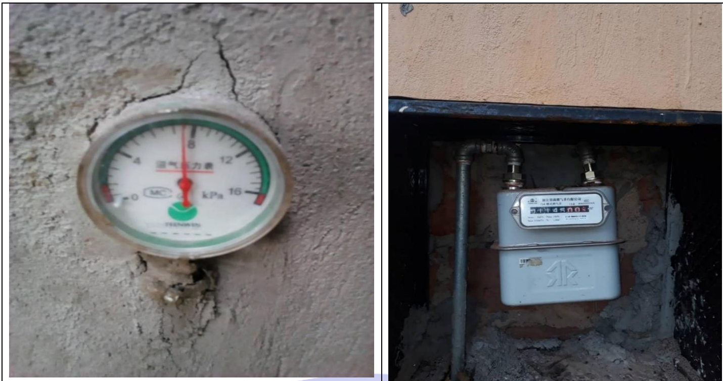
Installed gauges for monitoring pressure and gas levels
