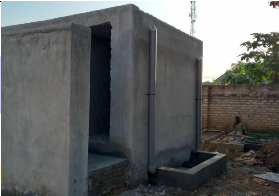
Construction of sustainable pit latrines with biodigester
